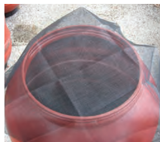
For barrels with a removable lid, unscrew the retainer ring and separate it from the inner lid, place screen over barrel opening, replace just the retainer ring to hold the screen in place, and trim excess screen material around the outside of retainer ring.
