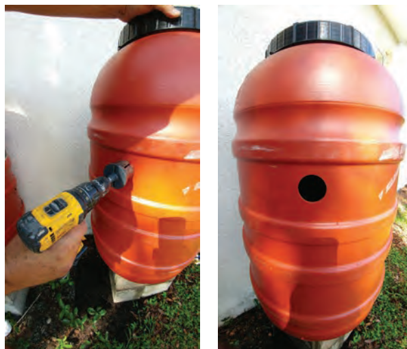
Drill a hole in each barrel for a connector. For a two-inch PVC male adapter, a 2-3/16-inch hole saw was used. Pick a flat spot on each barrel so connection is level.
