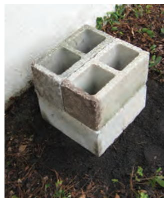
Stack blocks in a crisscross pattern for stable platform.
