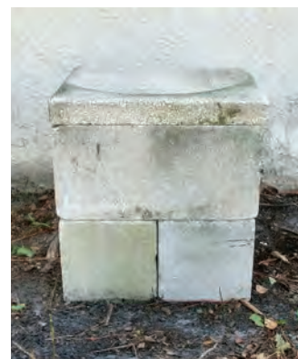
A flat paver stone can be placed on top of stacked block for added stability.
