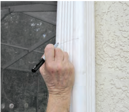
Based on the height of barrel, mark and cut the downspout, then securely attach the pipe or flexible downspout attachment with sheet metal screws or rivets.
