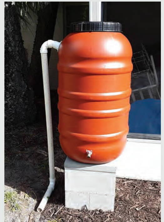
Slightly raising a rain barrel off the ground can help increase water pressure and provide easy access to spigot connections.
