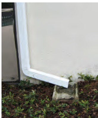
This spot will use an existing gutter and downspout.
