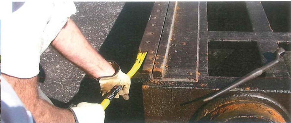
Remove Bottom Seal and Clamp Bar
