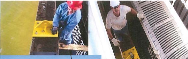
Attach Lift Plates to Bottom Half of Gate
