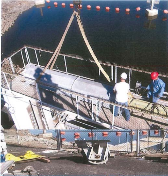
Remove Gate Lift Frame and Idler Sheave Hanger Frame
