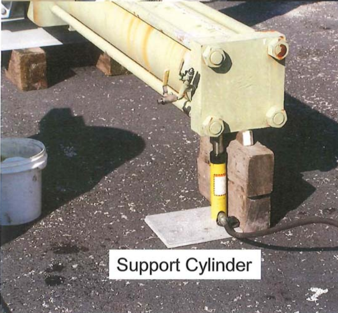
Remove Cylinder from Gate Hoist Frame
