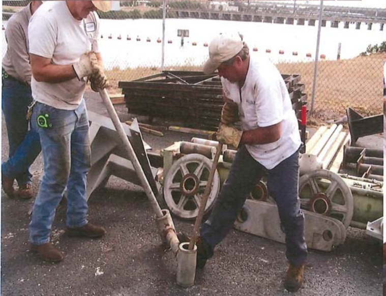
Disassemble Crosshead Sheave Assembly and Guide Rods
