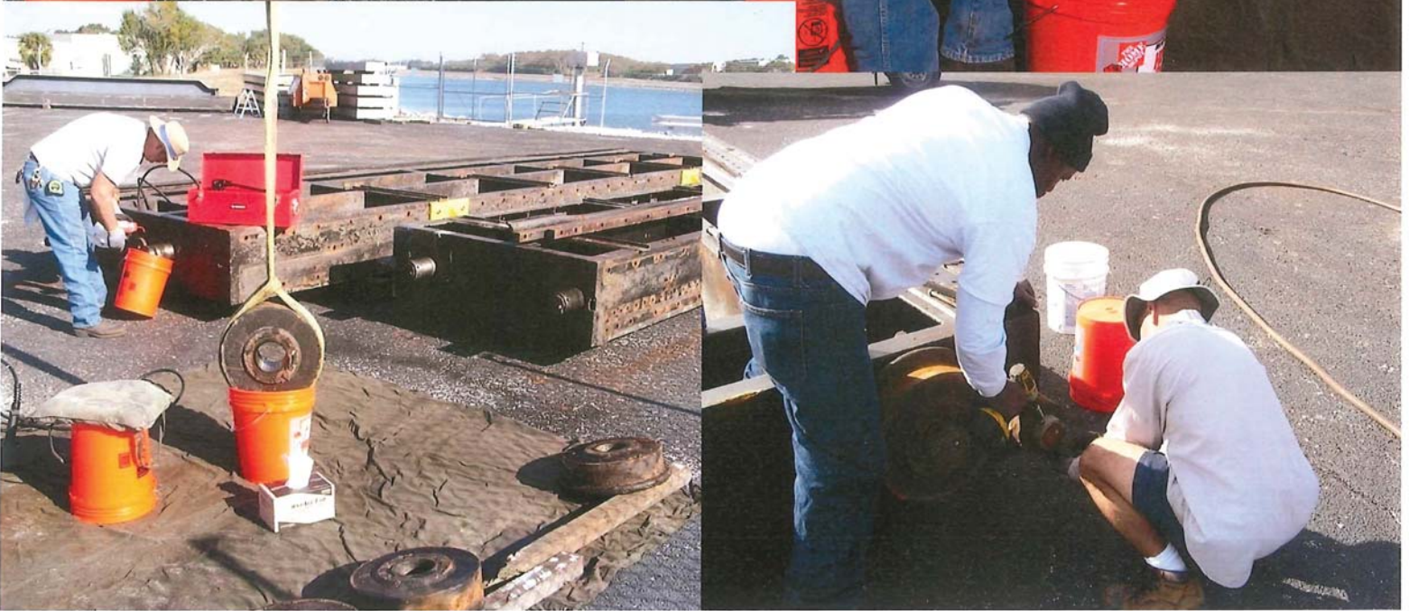
Remove Retainer Rings and Rollers
