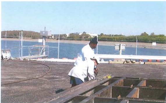
Remove Bottom Seal and Clamp Bar
