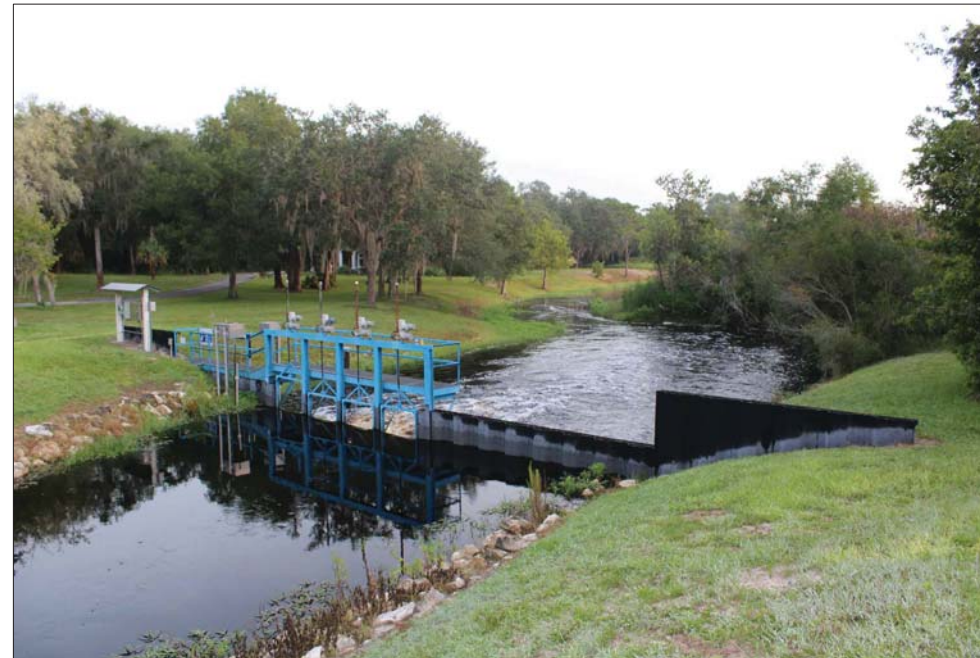
TSALA APOPKA GOLF COURSE STRUCTURE PHOTO (EXISTING CONDITIONS)
