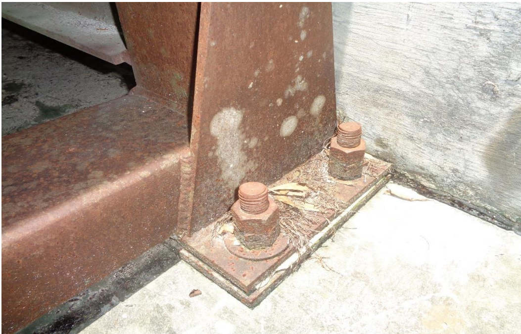
Photograph No. 11 – Typical Condition of Fasteners
