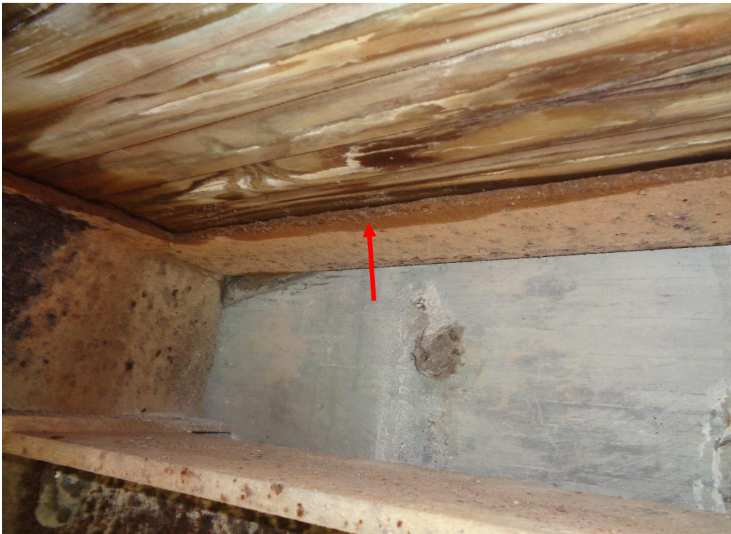
Photograph No. 7 – Corrosion of Top Flange Caused by Entrapment/Holding of Moisture by the Wooden Deck
