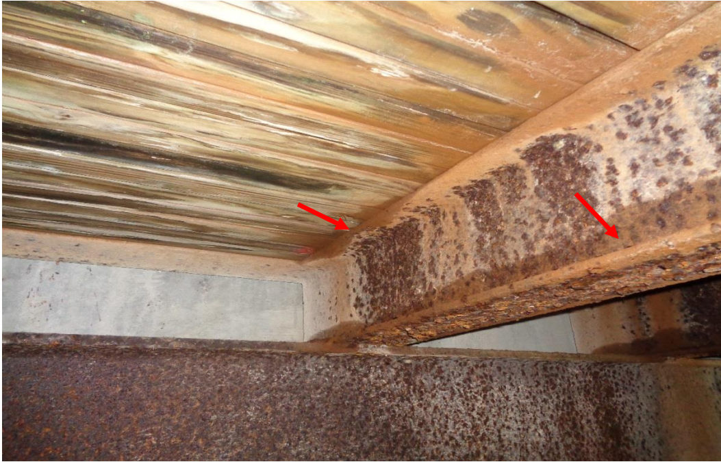
Photograph No. 10 – Moisture is Still Present Even Though Photo was Taken at the Peak of the Day Heat, approximately 2:00 pm
