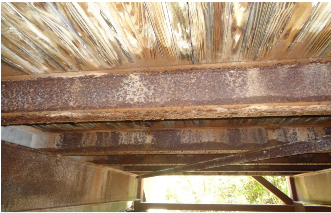
Photograph No. 5 – General View from Underneath Extensive Pitting
