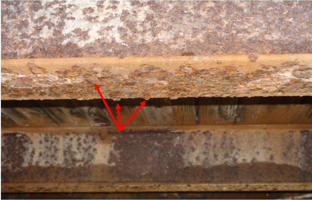
Photograph No. 8 - Rust Nodules on Bottom Flange Caused by Condensate
