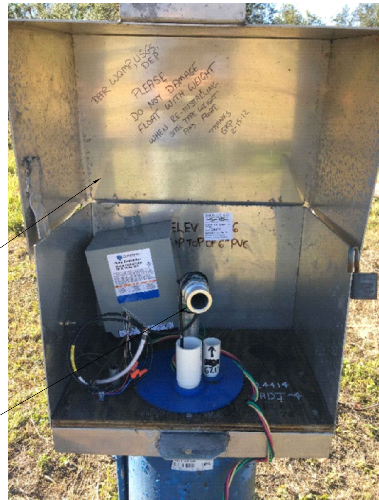
LOCKABLE WELL HEAD ENCLOSURE
