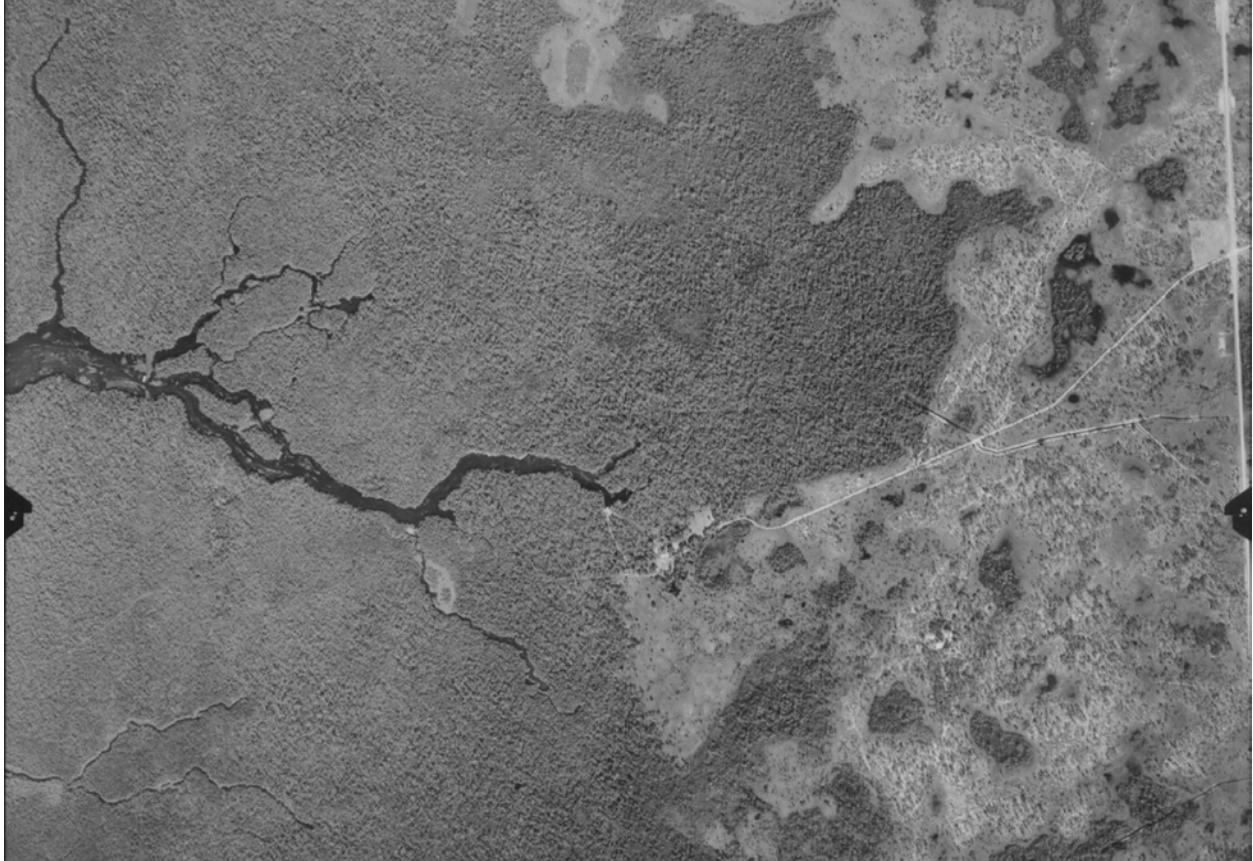
Figure 13: Historical aerial image of the upper Chassahowitzka River and surrounding lands from November 1944
