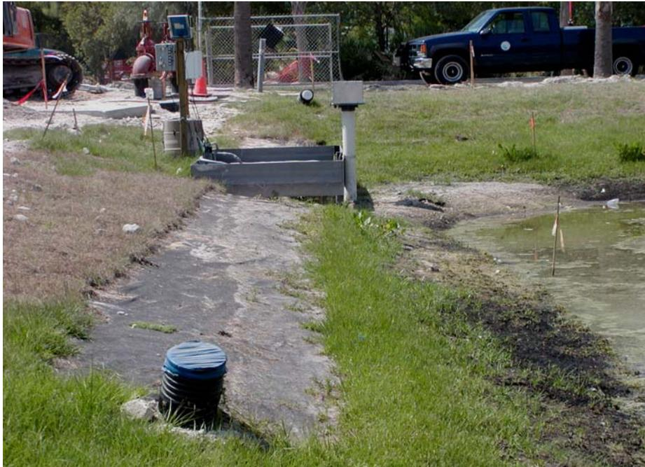
NORTH SIDE BANK FILTER COVERED TO KEEP FROM GETTING CLOGGED DURING CONSTRUCTION
