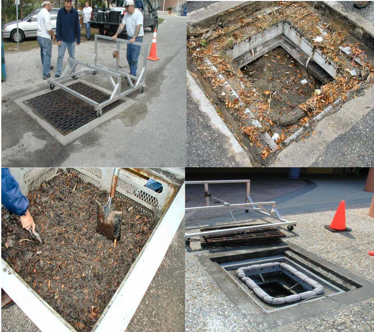
**Figure 26. Cleaning out the skimmer box inserts. a) Crane being moved into place to remove the grate. b) Uncovering the mess that is inside. c) Pushing all the material into the basket and mixing it well in preparation to taking samples to send to the lab. d) Installing cleaned out basket and new boom to make ready to replace the grate (photo credits: Suntree Technologies, Inc).**
