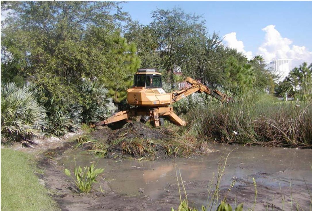
**Figure 34. Cleaning out bottom sediments and cattails in the Building pond during maintenance by Adopt-A-Pond.**
