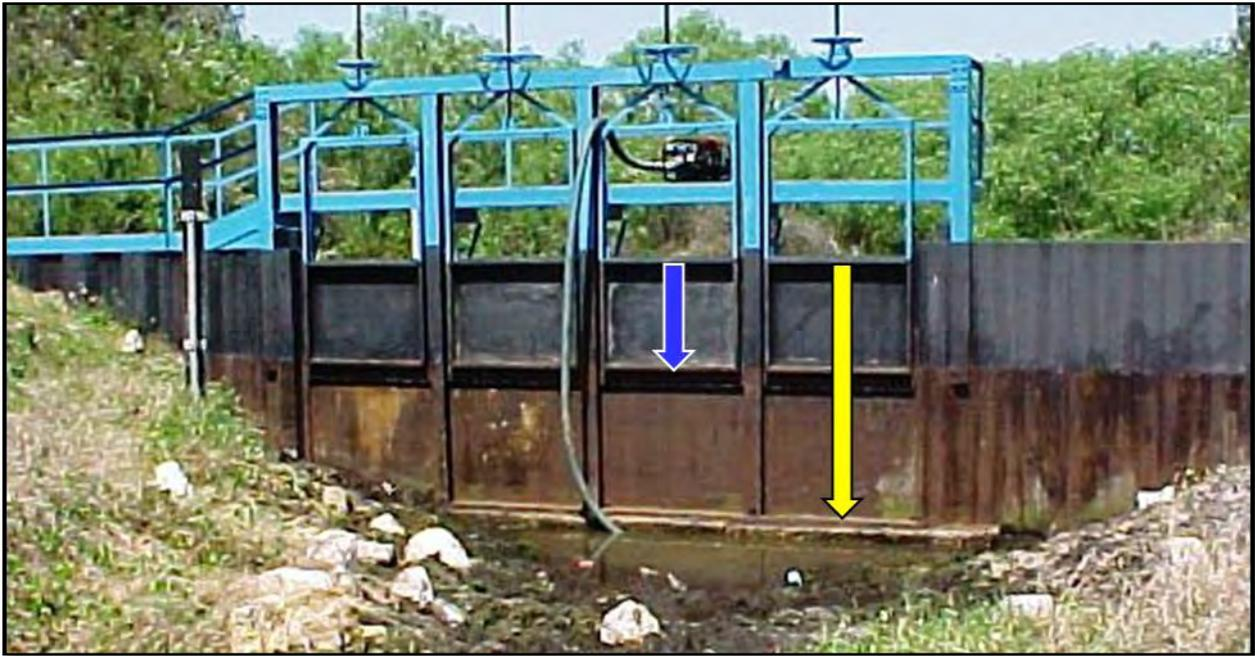
**Figure 13-2 Golf Course Structure with Existing and Simulated Gate Openings**
