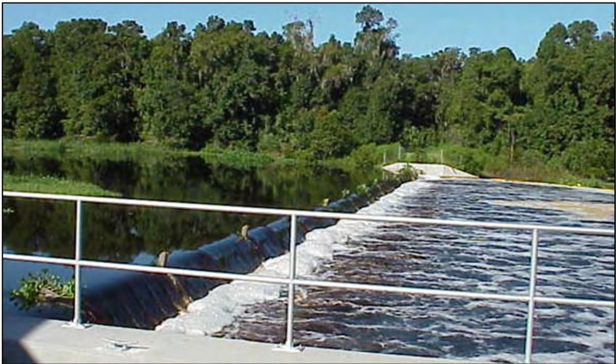
**Figure 7-3 Wysong Structure with Main Gate Fully Inflated (Raised)**
