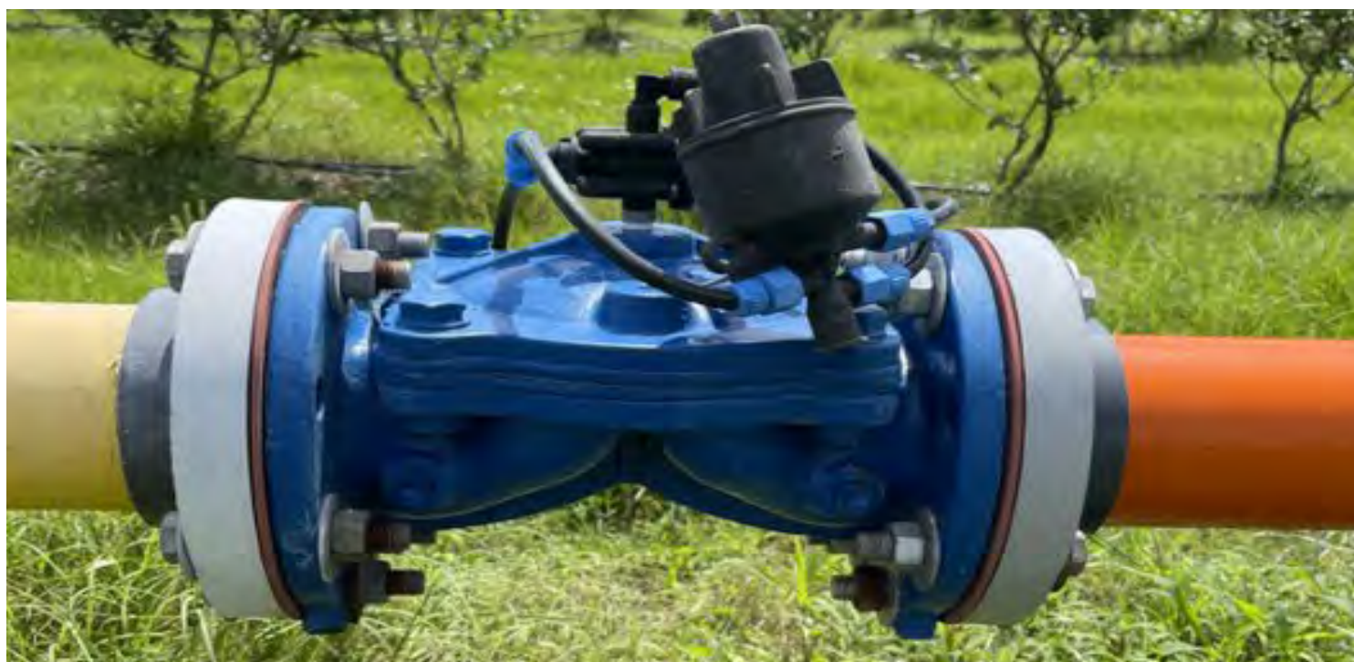
An electronic unit that can control irrigation system valves remotely and allow for reduced irrigation run times. Installed at M & R Blueberry Farm in DeSoto County through the FARMS program.
