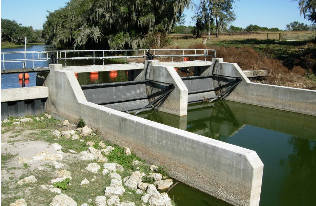
Figure 4. Downstream side of the former P-11 control structure showing two metal radial gates and the concrete-capped, sheet-pile wall
