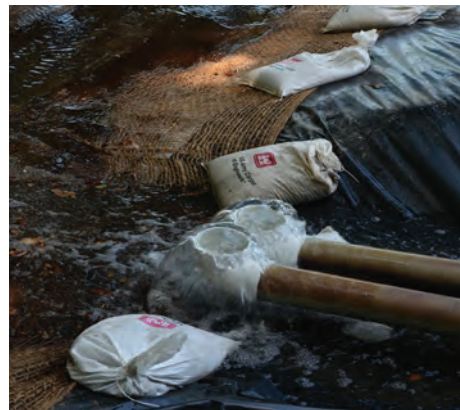
Water and muck slurry entering the dredge material management area at Lake Seminole.
