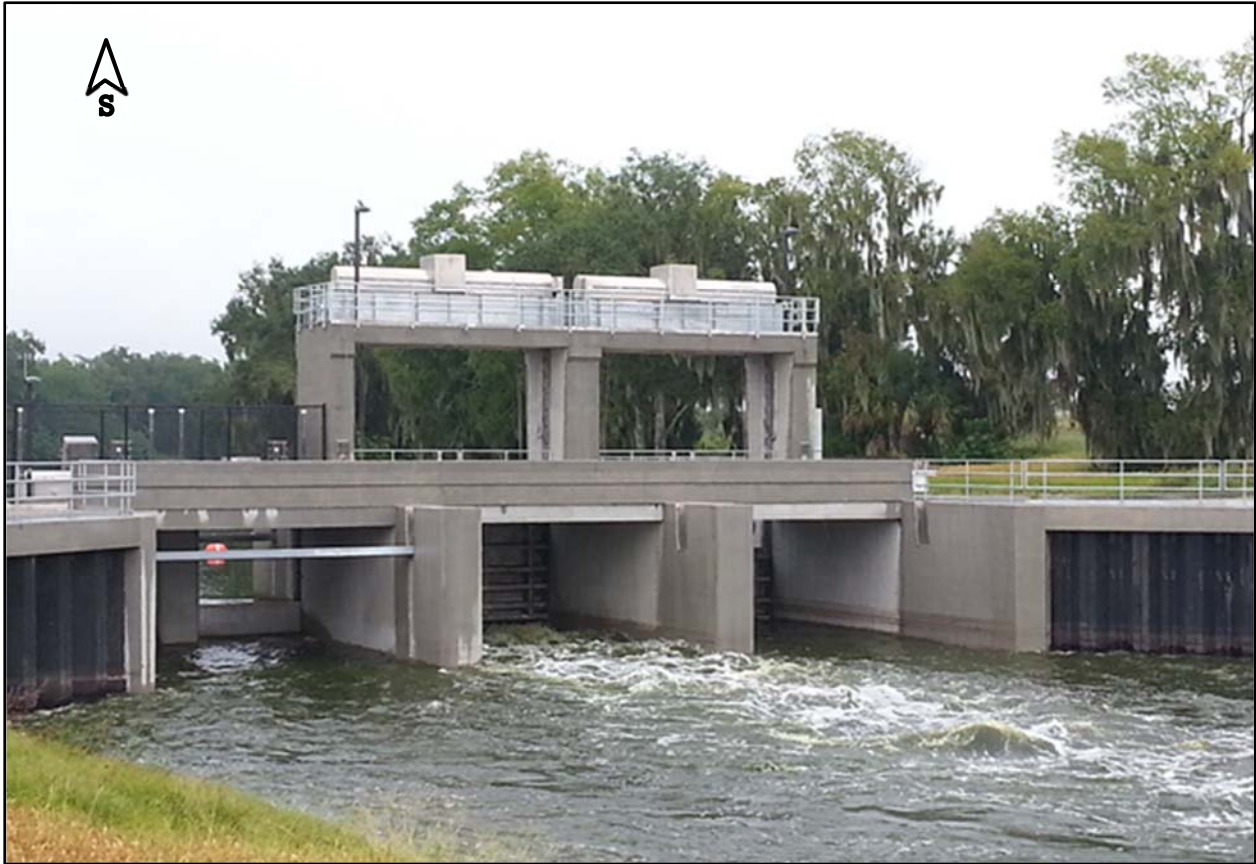
Figure 5. Downstream side of the Lake Hancock's P-11 control structure showing two weir gates in the westernmost bay on the left (one is partially open and the other is closed) and roller gates in the other two bays
