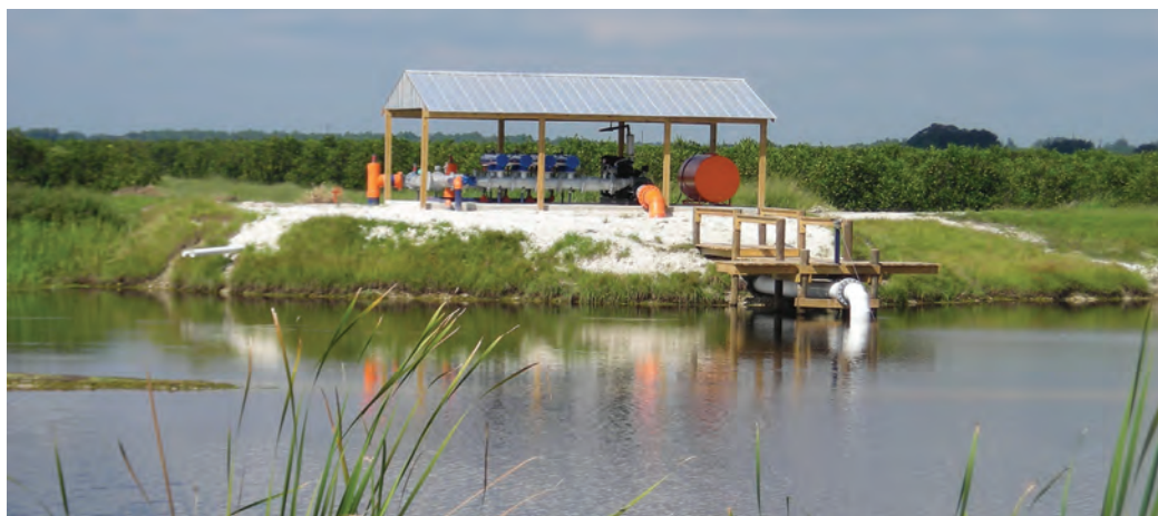
FARMS tailwater irrigation pumps.
