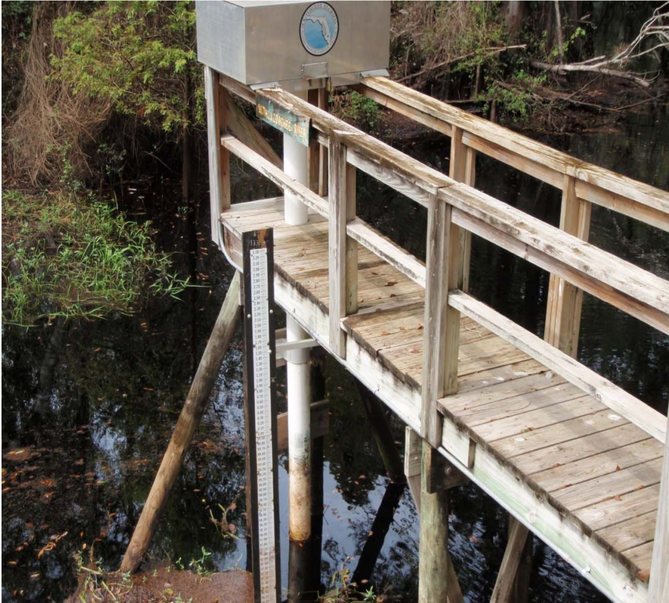
Figure 1: Stilling Well and Staff Gauge Facility
