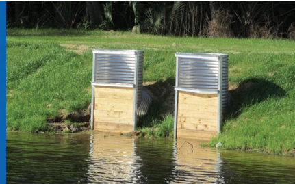
Riser Culverts and Water-Control Structures
