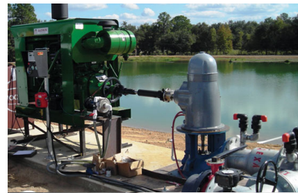
Surface Water Wet Well and Engine
