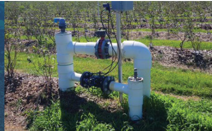
Remote Irrigation Zone Controls, and Soil Moisture and Climate Sensor Telemetry
