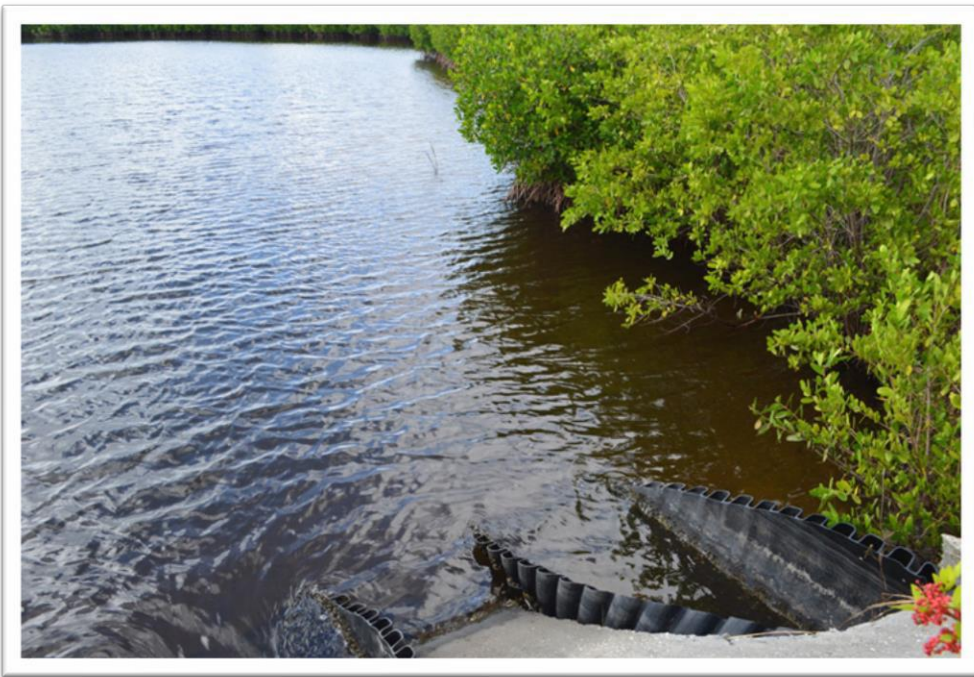
Cattle Dock showing culverts installed to reconnect tidal flows (2012)
