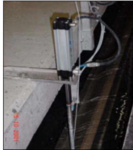
(Above) Automated pneumatic effluent weir actuator controls prescribed sludge removal cycle.
