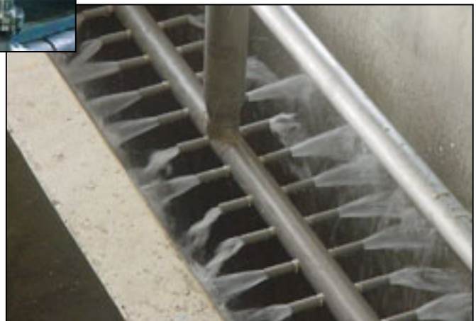
(Right) Rictor-type Air dispersion headers and nozzles
