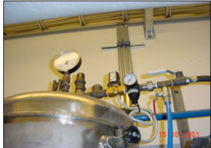
(Left & Below) A typical saturator vessel. Influent injector piece yields a high saturator efficiency, resulting in a small, compact saturator tank. All saturator MOC is 304 SS
