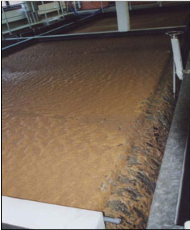
(Above) Automated pneumatic effluent weir actuator controls prescribed sludge removal cycle.
