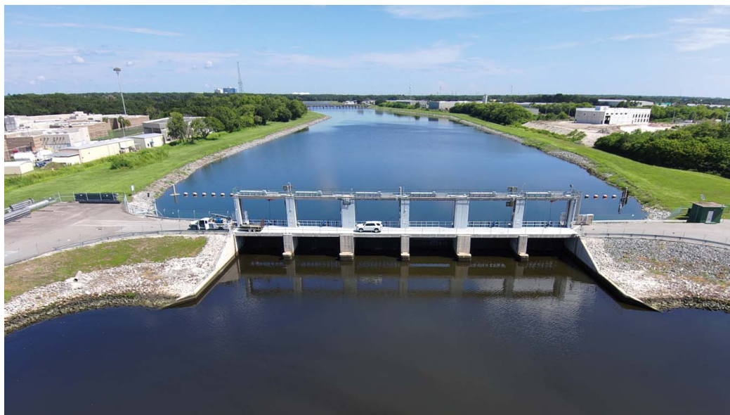
Tampa Bypass Canal.
