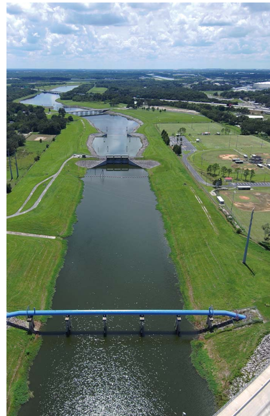
Tampa Bypass Canal in Hillsborough County.
