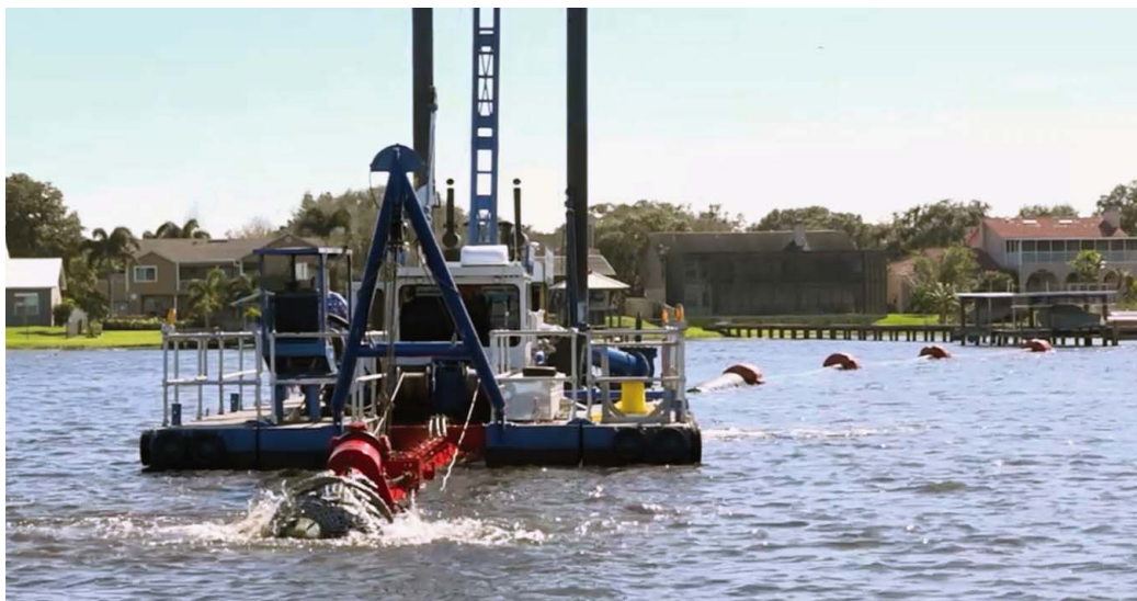
Dredging on Lake Seminole in Pinellas County.
