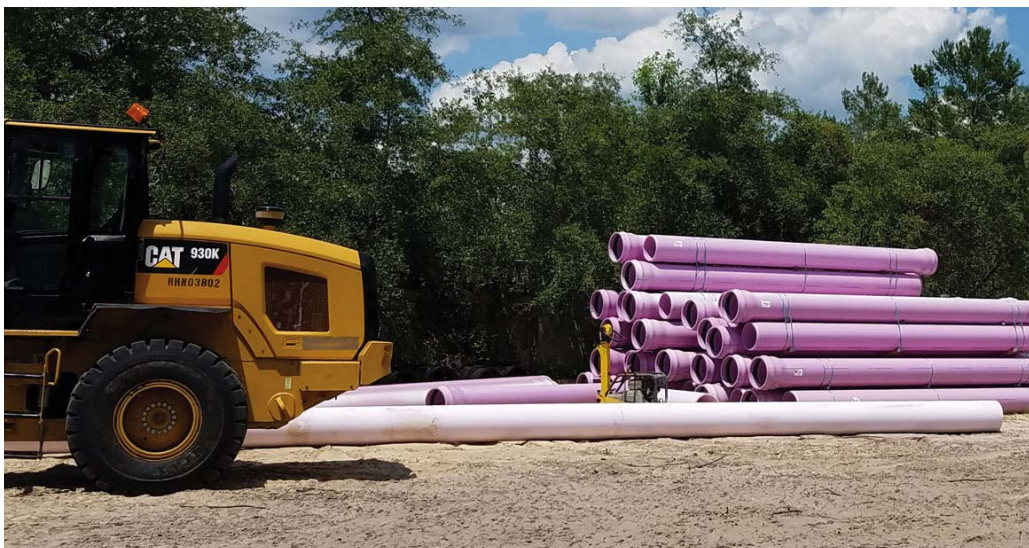
Reuse pipeline construction site.
