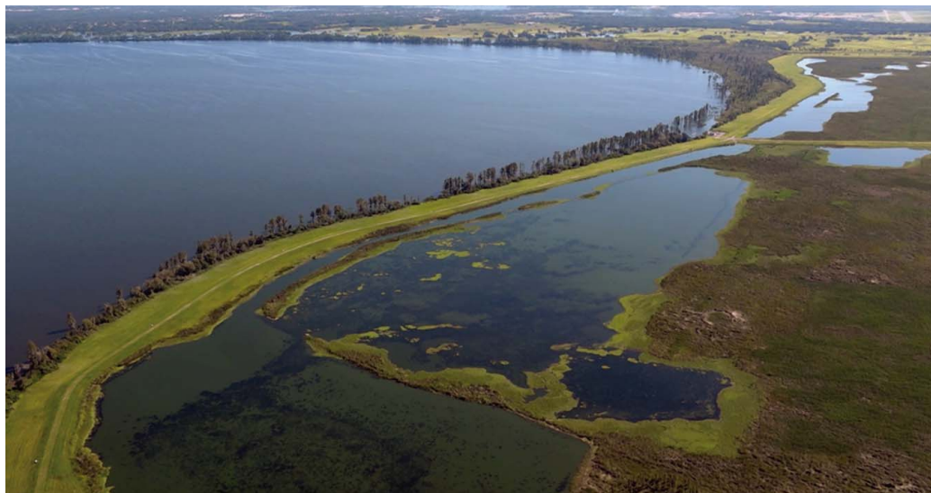
Lake Hancock Outfall Treatment System.
