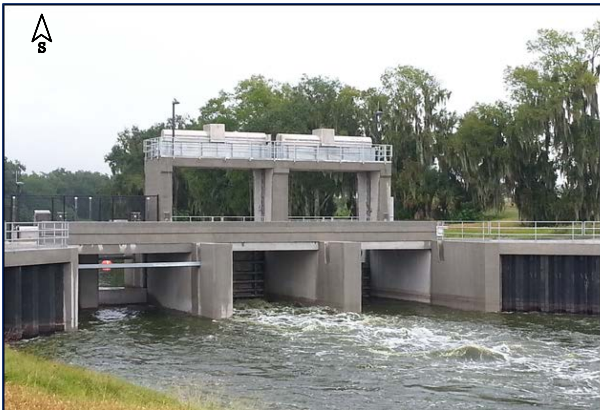
Figure 5. Downstream side of the Lake Hancock's P-11 control structure showing two weir gates in the westernmost bay on the left (one is partially open and the other is closed) and roller gates in the other two bays
