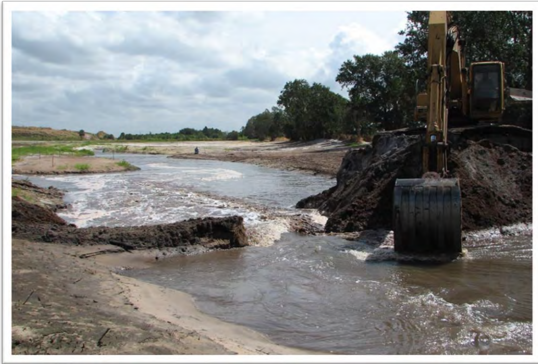
Marsh grades are final, and a backhoe breaches the canal block to open tidal connection and flow into the constructed wetland. (2005)
