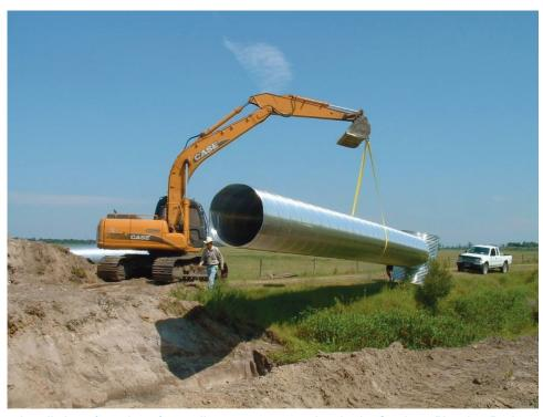
Installation of a culvert for a tailwater recovery project in the Southern Planning Region that will recover and reuse excess irrigation water. The District will provide funding for similar projects in the Northern Planning Region.
