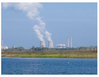
Progress Energy's Crystal River power station uses billions of gallons of salt water each day from the Gulf of Mexico for cooling purposes. The facility also uses much smaller quantities of fresh groundwater that could be reduced or replaced with reclaimed water from nearby communities.
