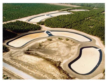
Highly treated reclaimed water produced in the Orlando area is piped to large rapid infiltration basins (RIBs) as part of the CONSERVE project. This type of water resource development project could be constructed in the Northern Planning Region to offset the potential impacts of groundwater withdrawals.
