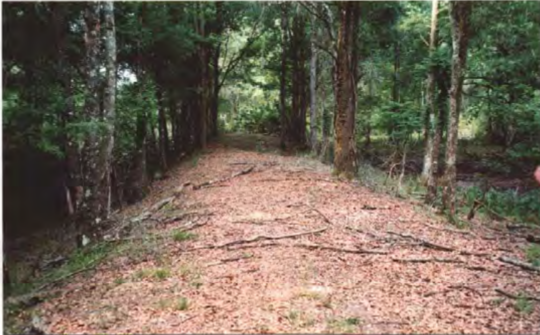
Site 4 – Portion of the abandoned tram berm north of the Pithlachascotee River. The berm breach will only be as wide as needed to restore flow (probably 30-40 feet) with gradual, stabilized slopes. Berm placement and construction will be located within an area to minimize removal of oaks along the sideslopes.
