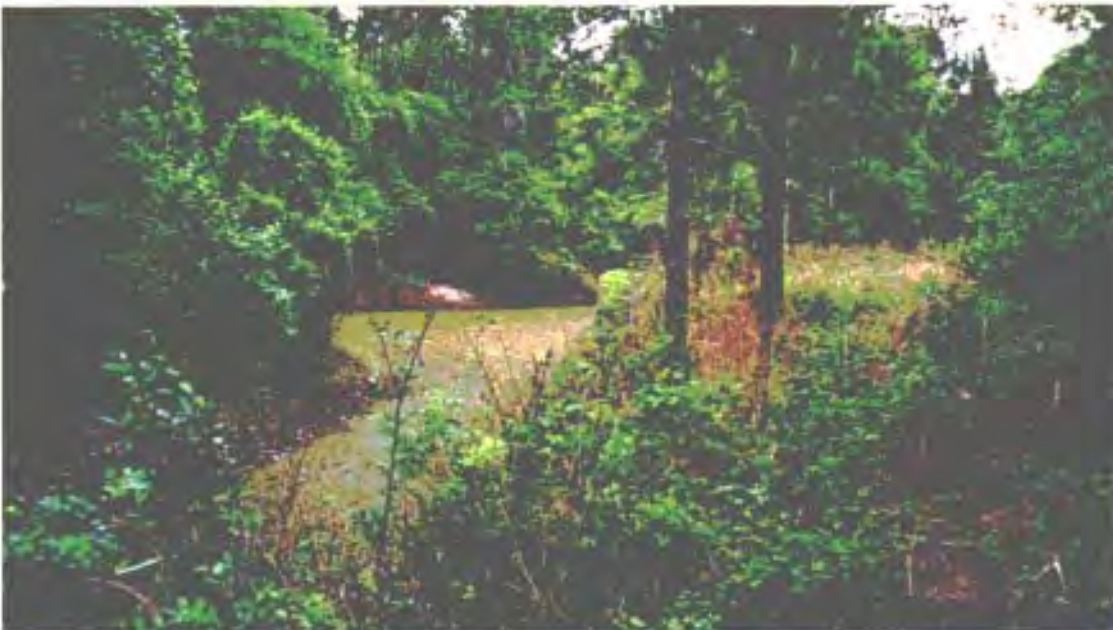
Sapling Drain – View from the spoil ridge of the Sapling Drain ditch (left) as it ties into the Gator Creek ditch (background). Spoil material will be backfilled into the drain to restore the wetland floodplain hydrology, and trees will be planted to aid in restoring the earthwork areas.
