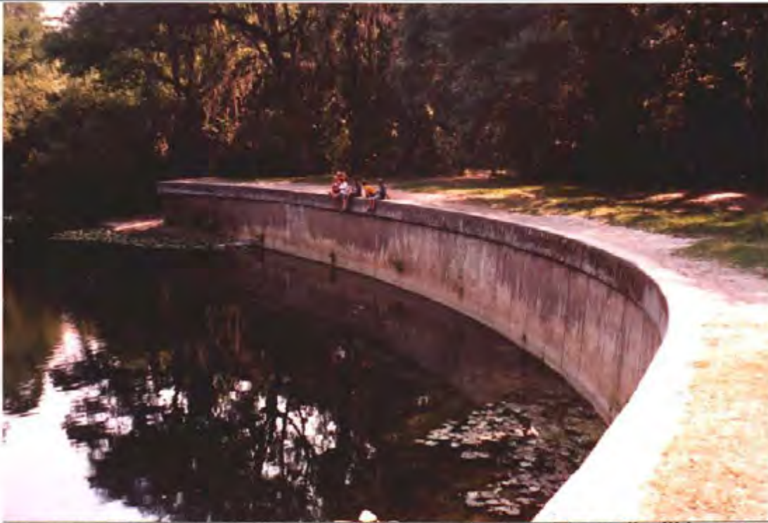
View of the bulkhead wall along the Hillsborough River. The wall will be removed and the area graded to reflect a more sideslope gradient, with tie-in to the grade elevation of the existing tree line (right). Native tree, shrub, and herb species will be planted to restore habitat function and value.
