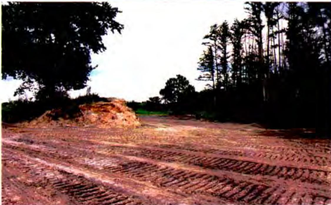
Same view as above photo after spoil material was backfilled. Preserved oak tree (left) on top of spoil mound depicts the amount of graded material required to fill the perimeter ditch.
