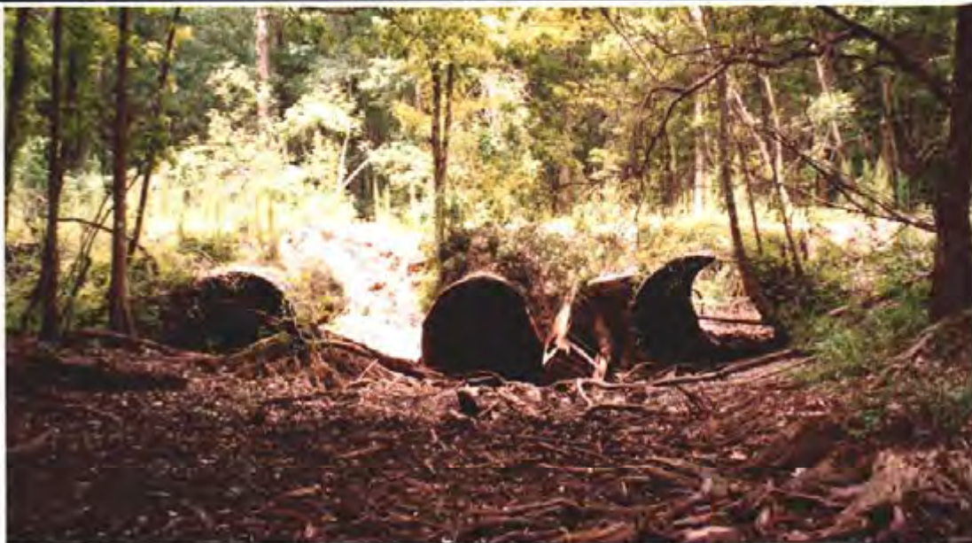
Site 2 – The undersized culverts within the main channel crossing of the Pithlachascotee River. Erosion evident between the center and left culvert, Abandoned refrigerator used as slope stabilization between center and right culvert. These culverts will be replaced with probably more and larger concrete culverts, as well as proper sideslope and pipe stabilization.
