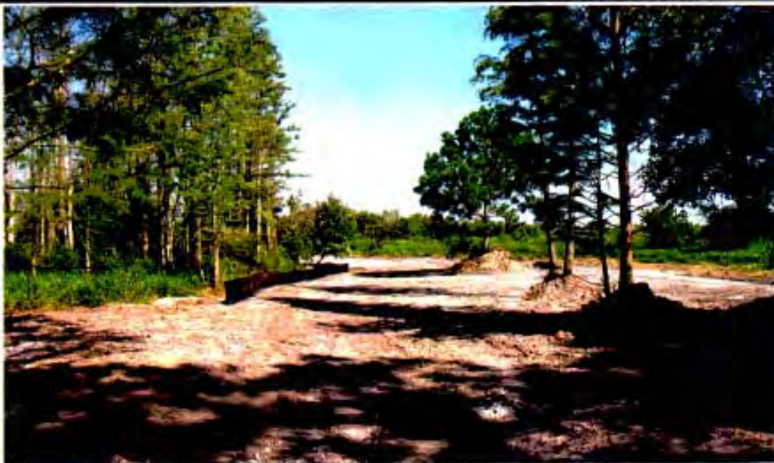
Same view as above photo after spoil material was backfilled. Silt screens installed to minimize erosion into the adjacent wetland while ground cover is establishing. Note where practical, construction worked around the drip line to preserve trees located on previous spoil ridge.
