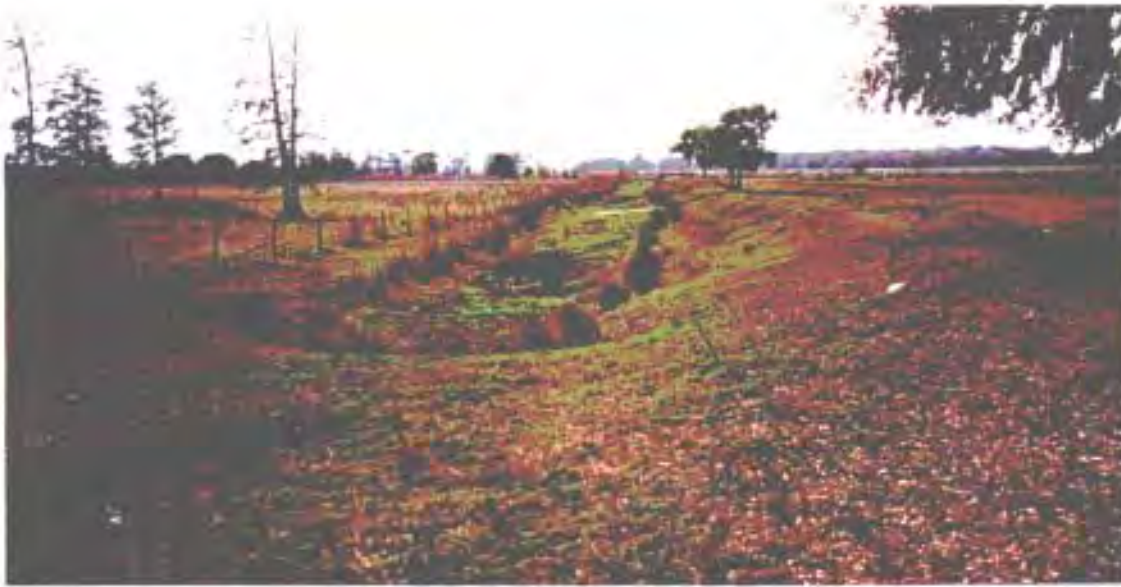
Central Access Road – View south along the access road berm to be reinforced (right) and adjacent ditch (center) that will be have ditchblocks installed to direct surface water flow to the northeast pasture (left and photo below).
