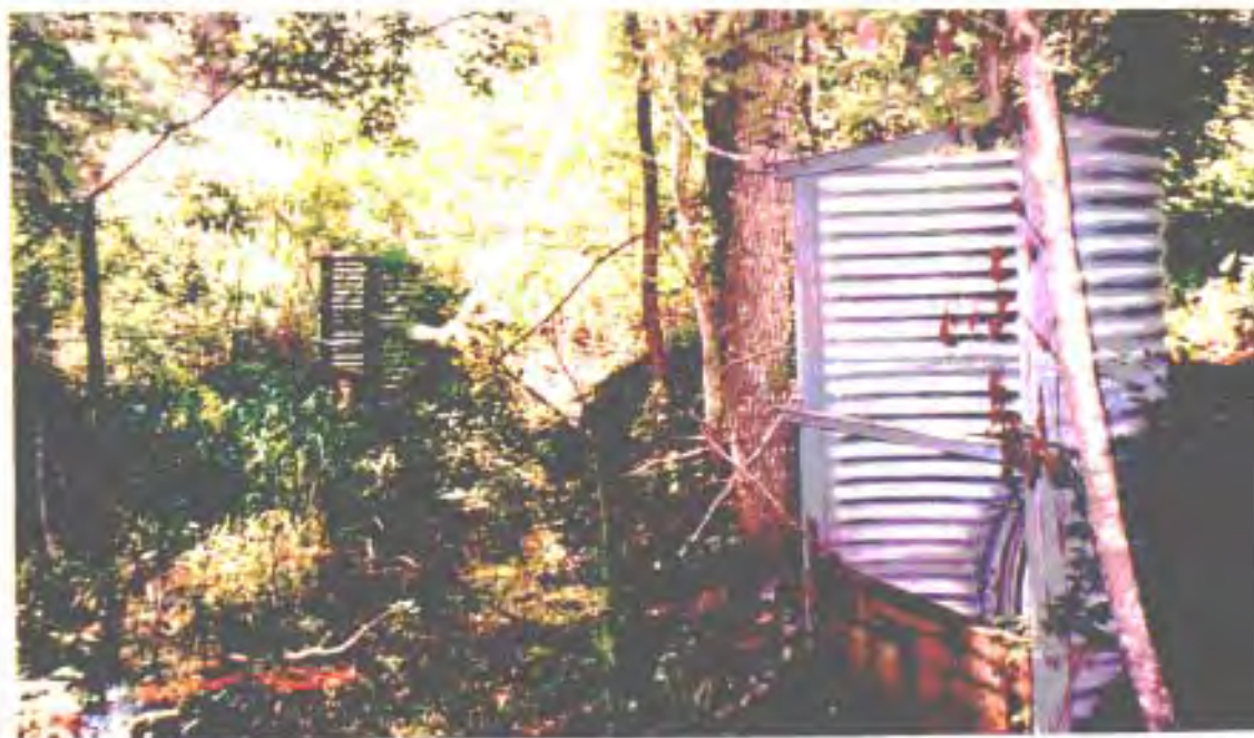
Photo 4 - The two outfall structures with flashboard risers that control the water elevation and flow from Ledwith Lake north to Levy Lake.
