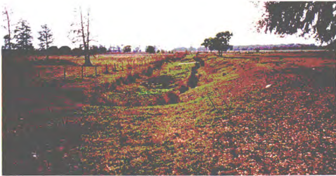
Central Access Road – View south along the access road berm to be reinforced (right) and adjacent ditch (center) that will have ditchblocks installed to direct surface water flow to the northeast pasture (left and photo below).
