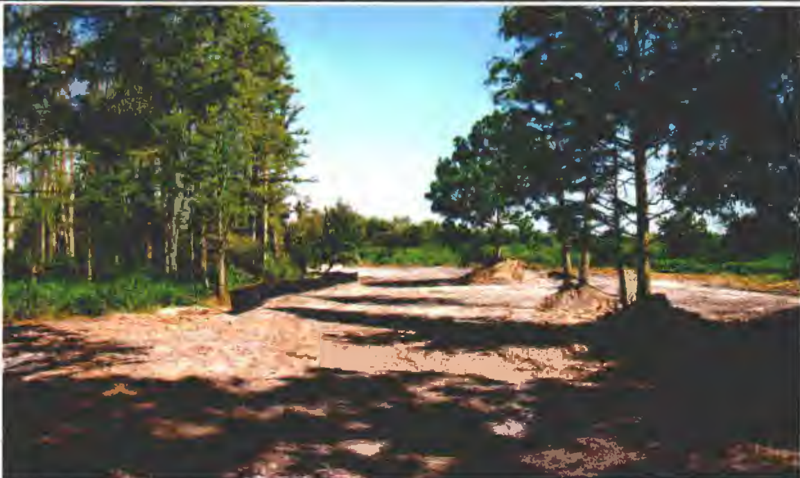
Same view as above photo after spoil material was backfilled. Silt screens installed to minimize erosion into the adjacent wetland while ground cover is establishing. Note where practical, construction worked around the drlp line to preserve trees located on previous spoil ridge.
