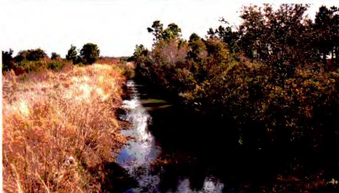
Photo 4 -View of the east-west ditch (15-20 ft. wide, 5-6 ft. deep) located through Wetland 2. Material to fill ditch will include existing spoil ridge (left, covered with broomsedge) and dredged material from the proposed cattle pond where the east-west ditch turns south. Existing vegetation (right) along top-of-bank will remain.
