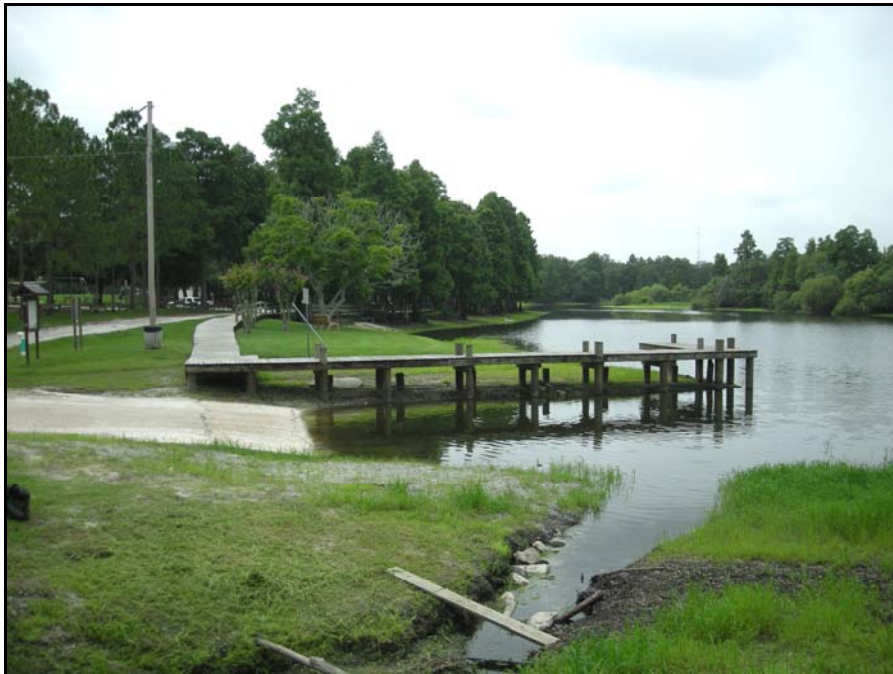
Figure 6-9. Photographs of public boat ramps and piers on the middle Hillsborough River at Rotary Park (upper panel) and Riverhills Park (lower panel) in June 2006 (District files).
