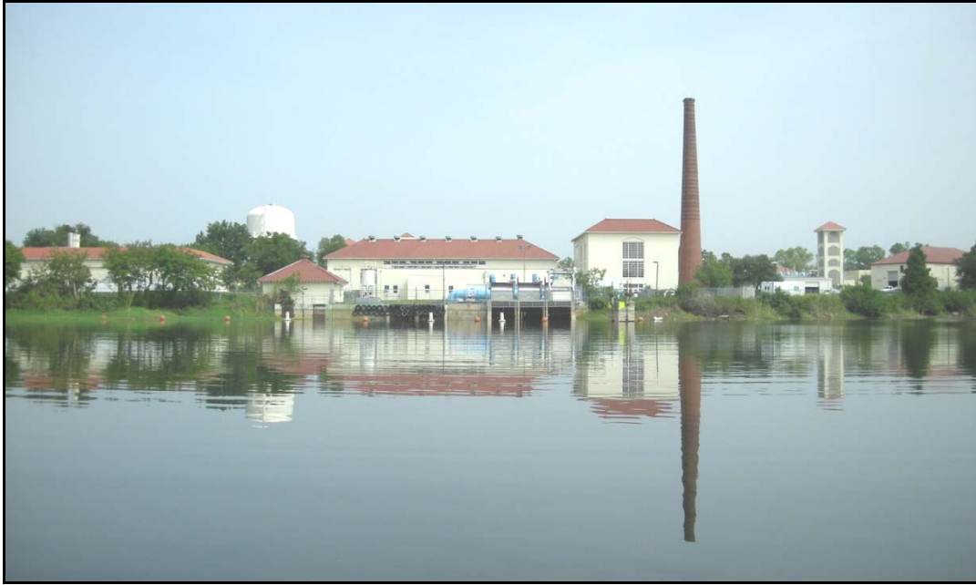
Figure 4-8. The City of Tampa David L. Tippin Water Treatment facility on the middle Hillsborough River (Southwest Florida Water Management District files).
