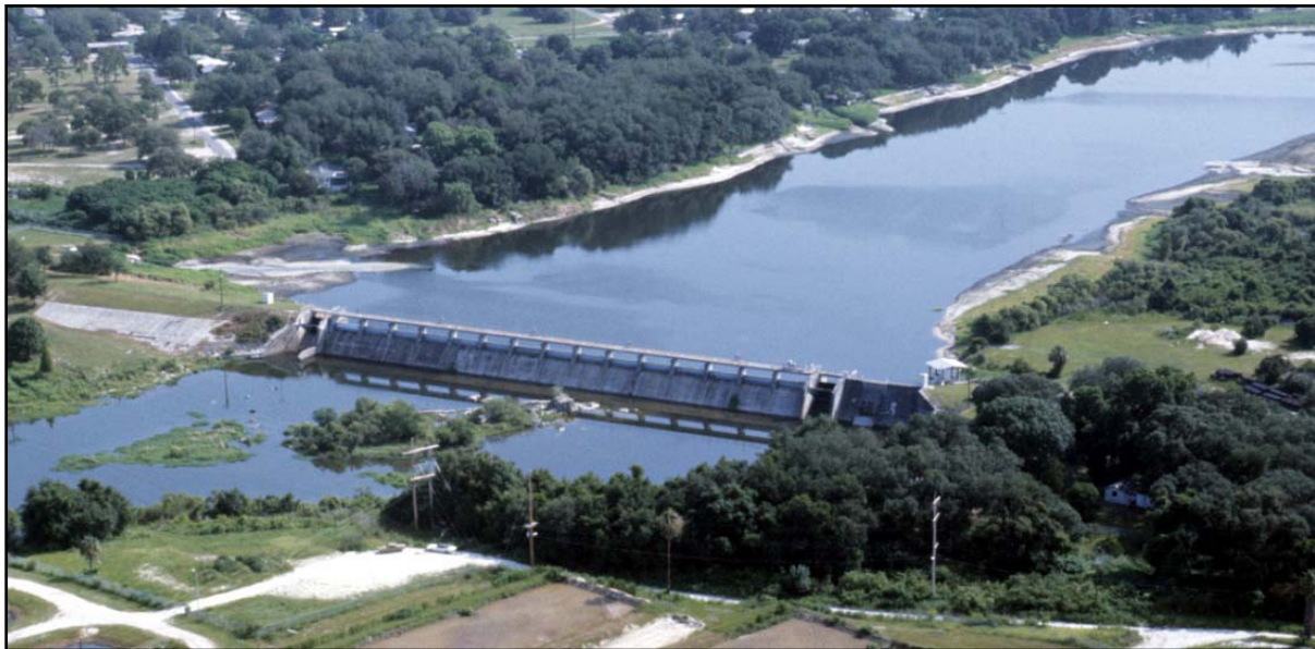
Figure 2-5. Aerial photographs of the City of Tampa Dam on the Hillsborough River. Upper photograph is from 2000, date unknown for the lower photograph (Southwest Florida Water Management District files).
