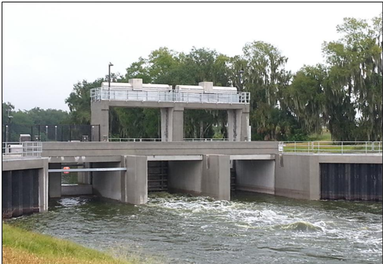
Figure 2-40. Downstream view of the Lake Hancock P-11 control structure, showing two weir gates in the leftmost bay (one partially open and one closed) and roller gates in the other two bays. Adopted from Yang et al. (2020).
