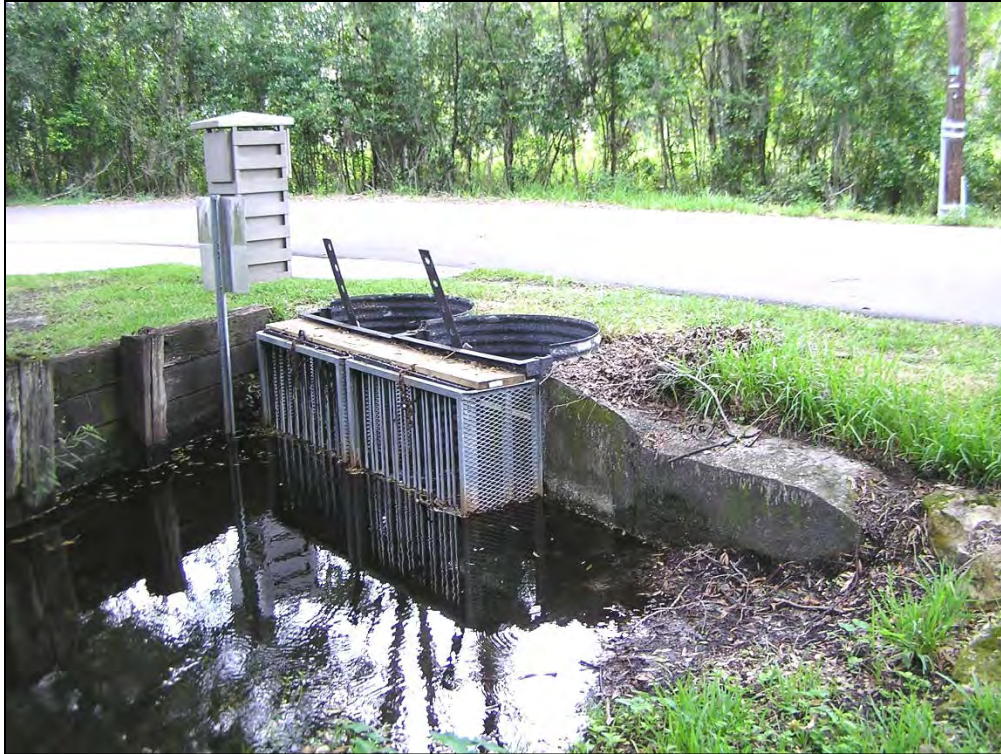
Figure 16. Operable structure installed on the outlet of Saddleback Lake.
