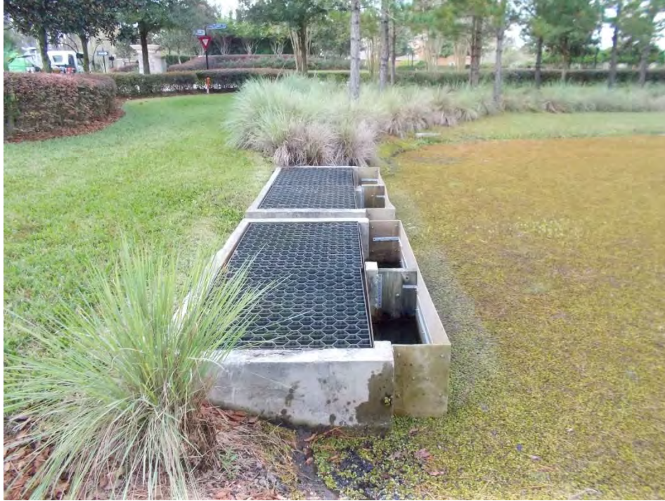
Figure 4: Two inflow weirs receive water from Reinheimer Lake under Van Dyke Road.
