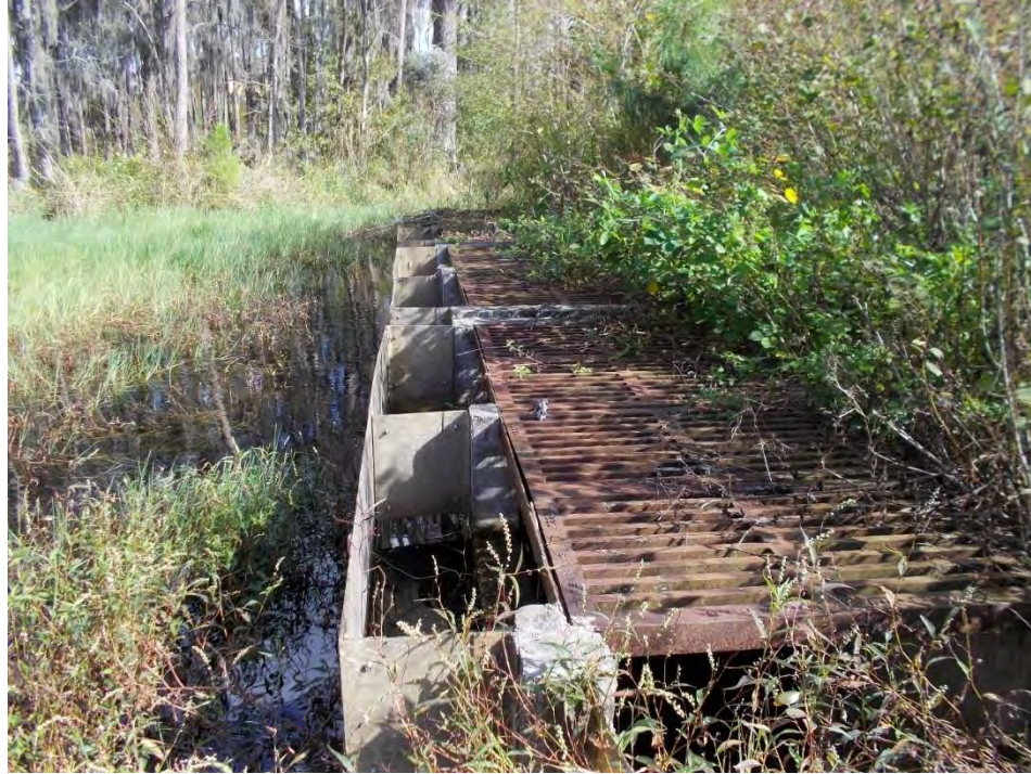
Figure 6: Three outflow weirs that serve as the control point out of the lake.
