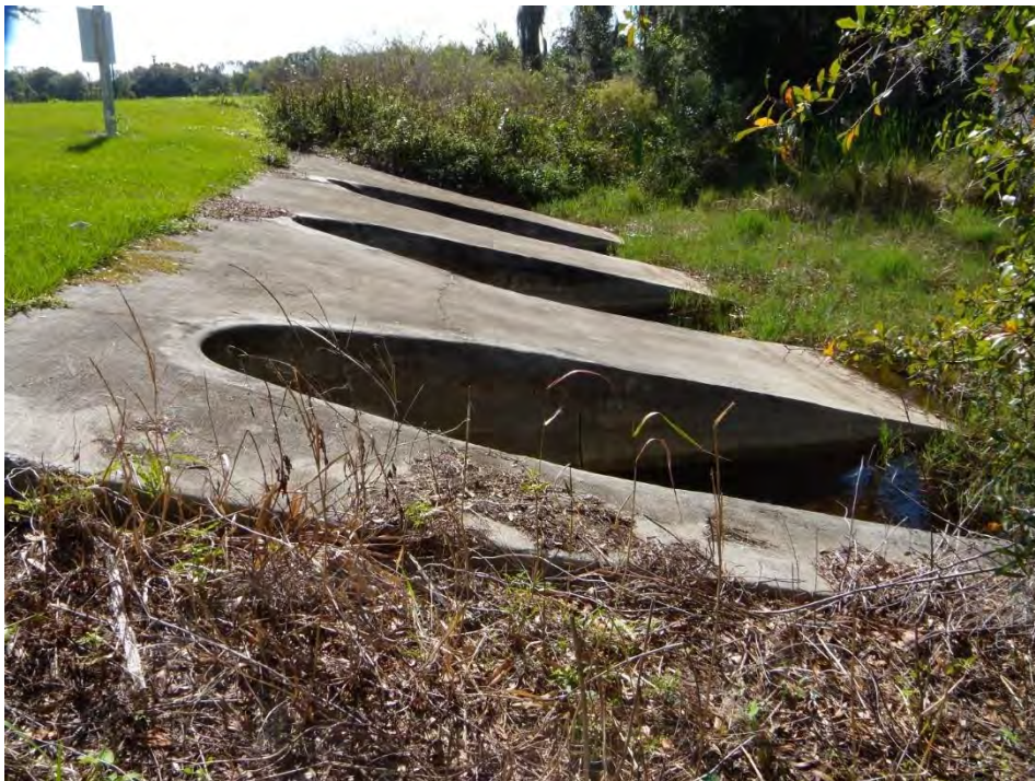
Figure 5: Four 60"X38" culverts under Merrywater Drive serve as outflow from the lake.
