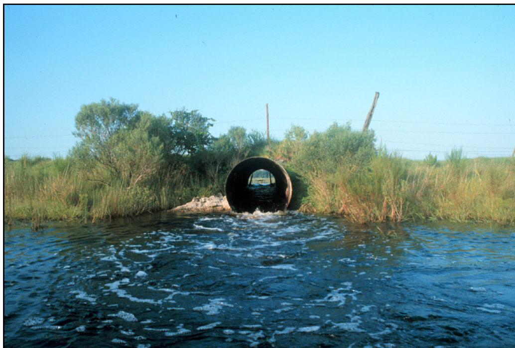
Figure 6. Photographs of the earthen berm that separates the northern and southern sub-basins of Crews Lake and the culvert that provides for surface water conveyance past the berm. The upper photograph, from 1971 (District files), also shows a portion of a secondary berm in the northern sub-basin that partitions a portion of the sub-basin from the rest of the sub-basin. The lower photograph shows flow between the northern and southern sub-basins in 1982 (District files).
