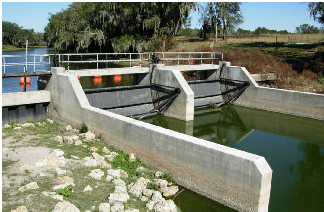
Figure 4. Downstream side of the former P-11 control structure showing two metal radial gates and the concrete-capped, sheet-pile wall
