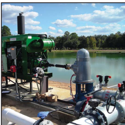
Surface Water Wet Well and Engine
