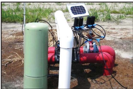
Remote Irrigation Zone Controls, and Soil Moisture and Climate Sensor Telemetry
