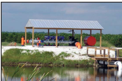
Surface Water or Tailwater Irrigation Pumps and Filters
