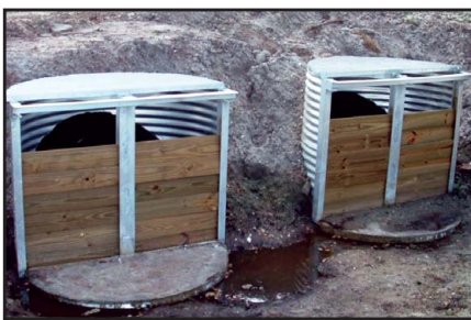
Riser Culverts and Water-Control Structures
