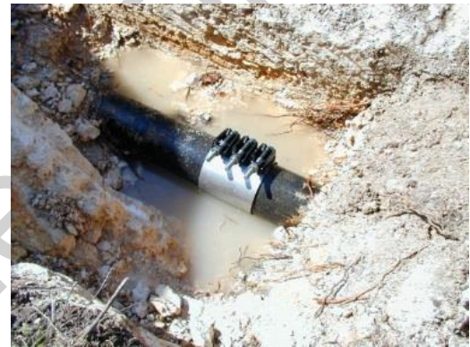
Repaired water main. The District performs leak detection surveys to reduce water loss.
