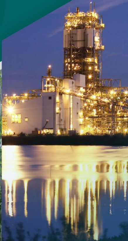
TECO Power Station Polk County
