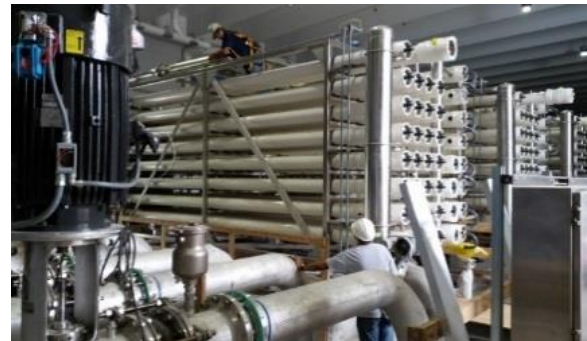
RO systems use high pressure and semi-permeable membranes to desalinate seawater
