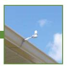
These devices override the system when enough rain has fallen or the soil is moist enough to skip an irrigation cycle.
