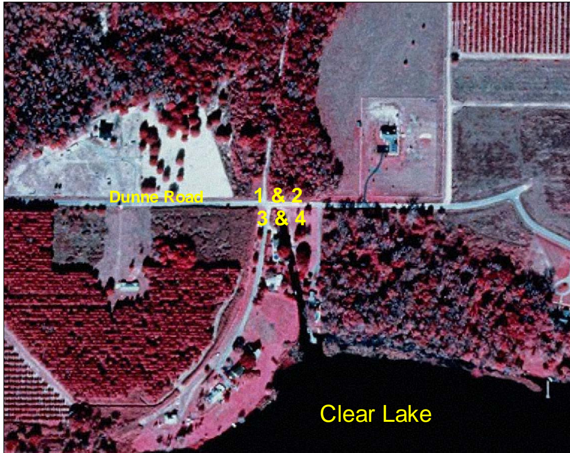
Figure 7. Outlet conveyance system for Clear Lake in Pasco County, Florida.
