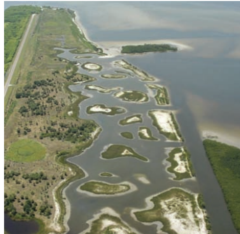
Aerial view of the Fred and Ida Schultz Preserve, a SWIM Tampa Bay Restoration project.
