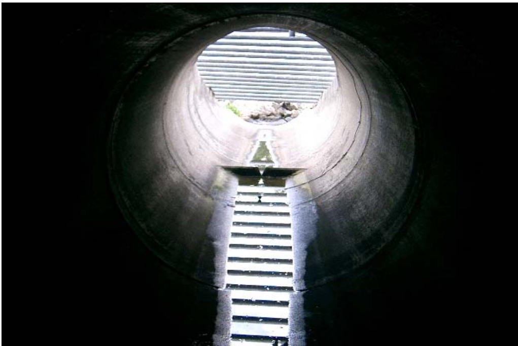
Inside the pipe looking out toward the pond. The base flow weir is shown.
