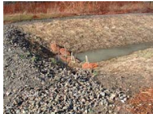
Swale and Gravel Filter Dam
