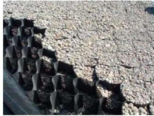
Gravel Storage Area Construction
