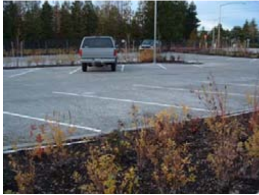
Porous Concrete Parking Lot
