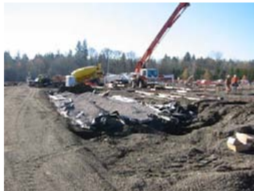
Gravel Coverage During Construction
