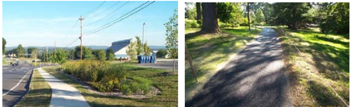
Porous Concrete Sidewalks and Porous Asphalt Paths
