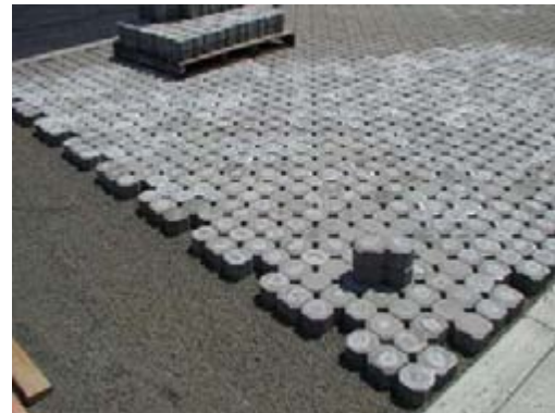
Paver Block Construction
