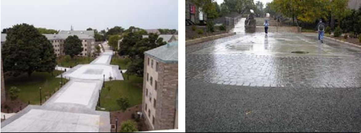
Plaza w/ Porous Concrete Strip at Villanova University (right side: during rain)
