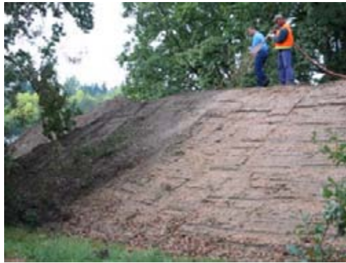
Spraying Erosion Membrane
