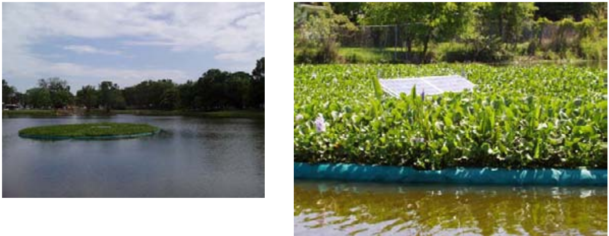
Figure 1. The floating wetland deployed in Lake June. The photo on the right depicts a closer view of the solar panels and vegetation.
